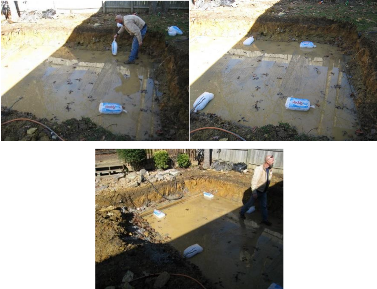
Figure 7. Ice Bag Positioning in Excavation
